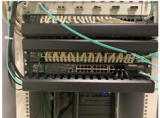
PoE Switch delivers power to APs
